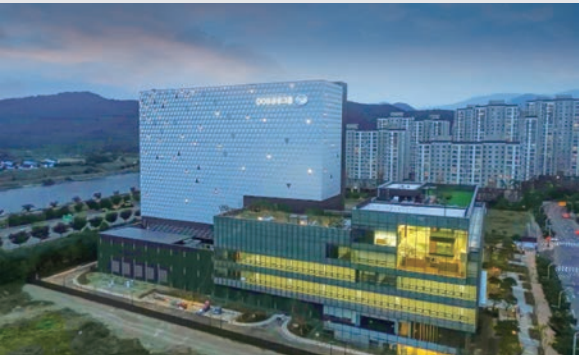
Daegu Bank (DGB) Data Center
