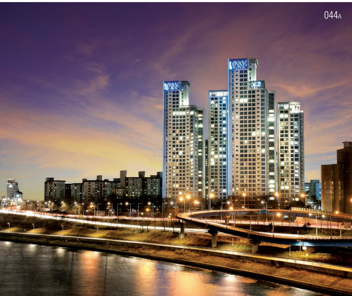
043A Misa Gangbyeon Central Xi Location: Hanam, Korea - Housing units: 1,222 Project period: 2014. 10 ~ 2017. 02
