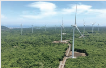
Onshore Wind Power (Jeju Gimnyeong Wind Power Complex)
